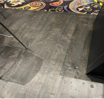
For rollable vinyl, place ½" plywood between the ¼" padding and rollable vinyl to create a solid subfloor
